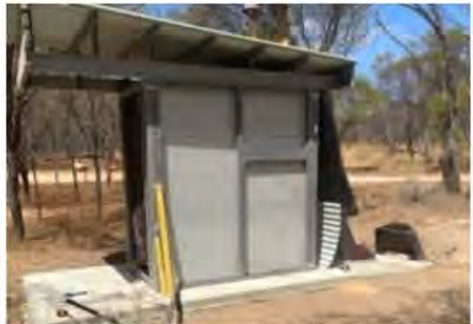
Above: Installing toilet at Jam Patch
