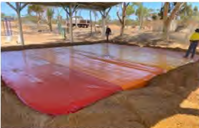
Above: Installation of Jumping Pillow at Newdegate Sporting Precinct.
