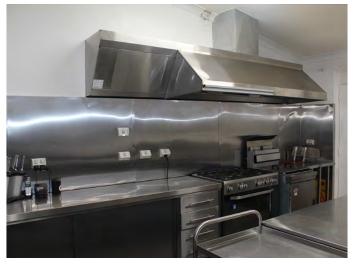
Below: New stainless steel splashbacks and modified range hood.
