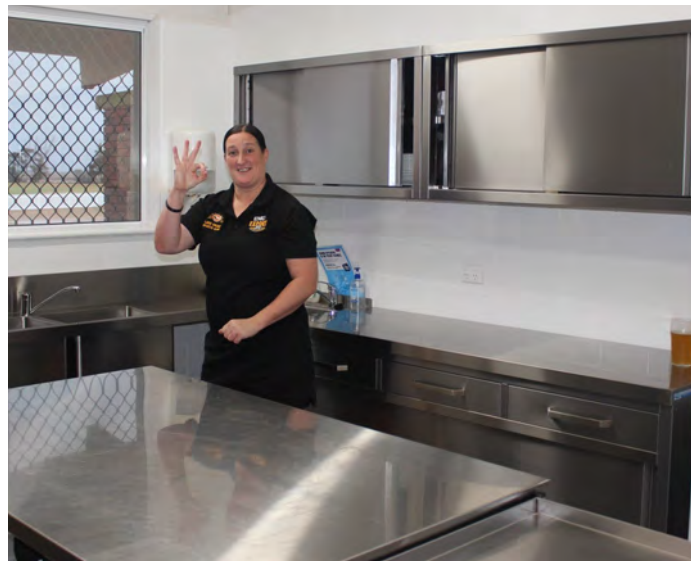
Below: New stainless steel splashbacks and modified range hood.
