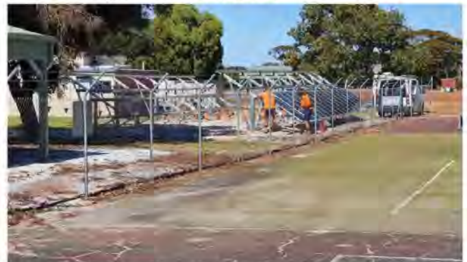
Above: Solar panels going in at Lake Grace Swimming Pool
