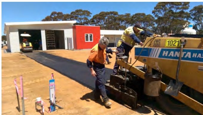
Asphalt being laid in front of new ambulance building.
