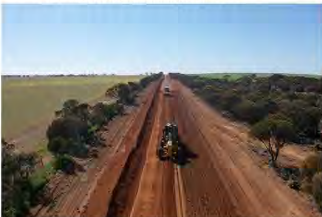
Above: Preparation of Mallee Hill Road
